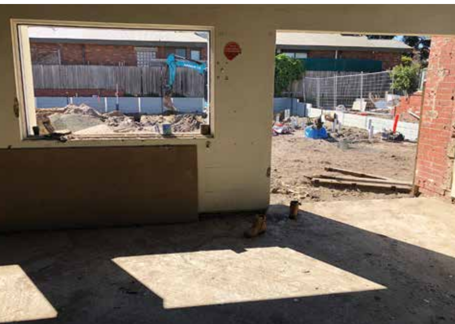
VISION: LOOKING OUT TOWARDS THE NEW BUILDING ADDITION.
