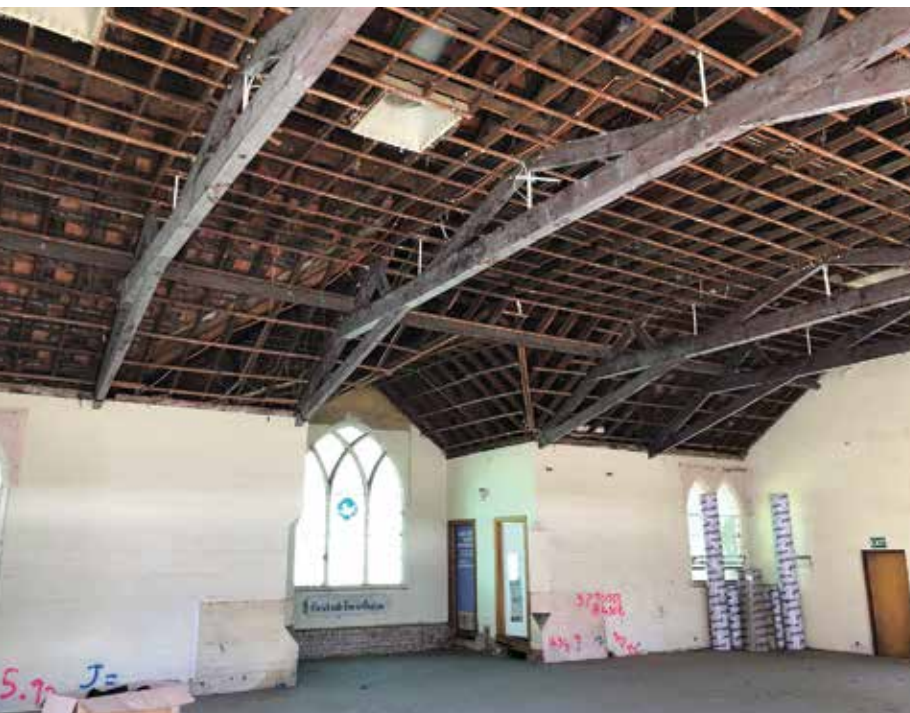
TRADITION: THE FORMER CHURCH SANCTUARY IS BEING TRANSFORMED.
